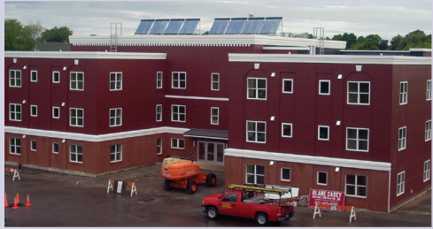
Market Square Commons in Houlton, a 28-unit senior housing development. Market Square is the first affordable housing development in Aroostook County in 15 years.
