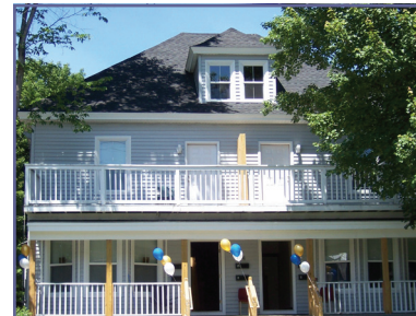
44 Fairfield Street in Oakland, providing 6 units of housing to people who were homeless.
