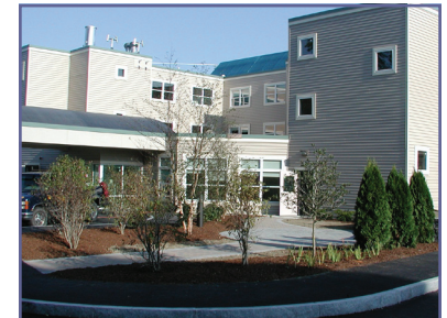
Pleasant Crossing in Waterville, providing 21 units of affordable housing to area senior residents.
