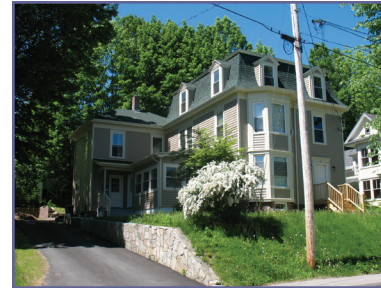
Washington Street Transitional Housing in Rumford, providing 2 units of housing for people who were homeless.
