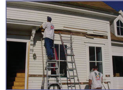
In 2009-10 MaineHousing invested nearly $2 million of HOME Fund money in home repairs and nearly $1 million in weatherization. Both improve Maine's housing and create jobs for Maine workers.
