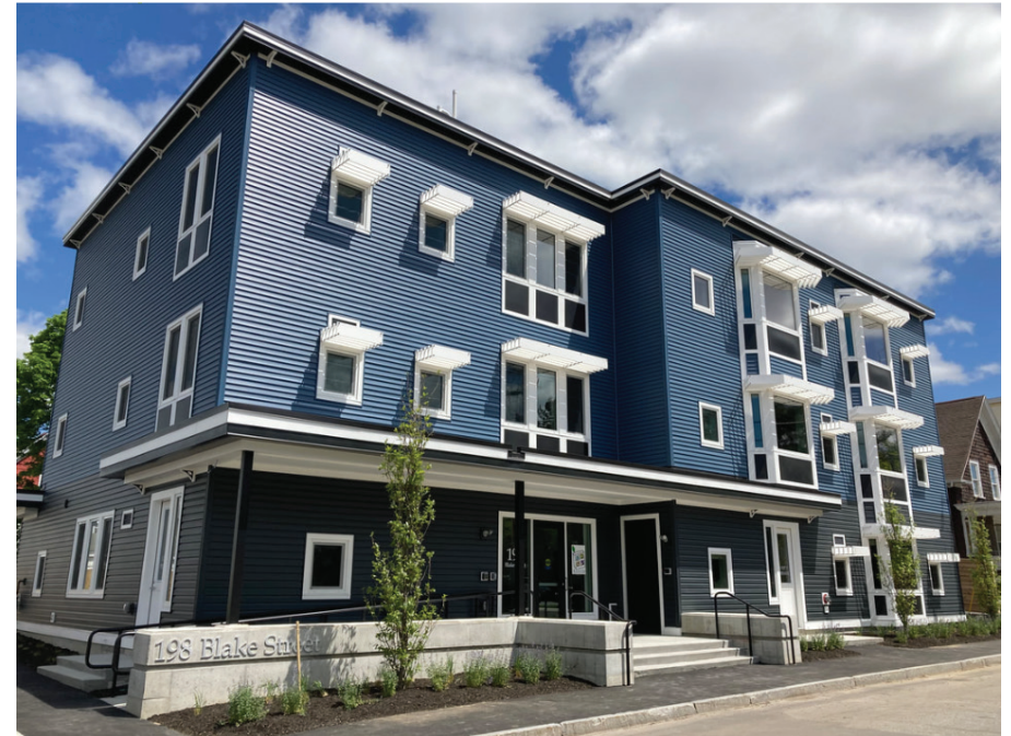
Blake & Walnut, two identical apartment buildings built in the style of the classic New England triple decker, located in the Tree Street Neighborhood of Lewiston. The buildings contain 18 new construction units for families, funded in part by the State HOME Fund.
